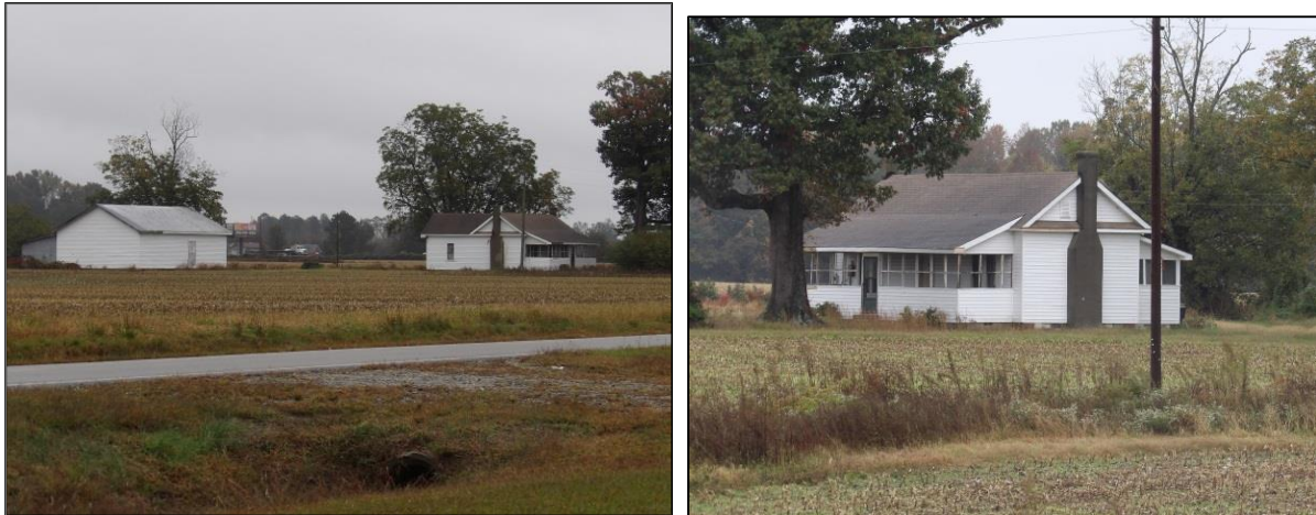
Photo 34: House, 5204 Ringwood Road, Southwest Oblique (Left) and Southeast Oblique (Right).
