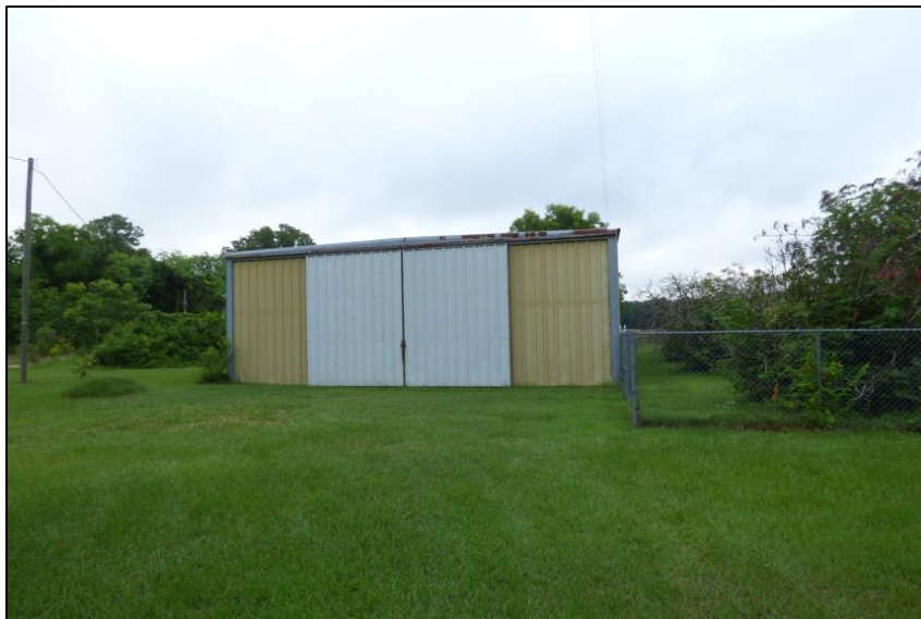
Photo 46: Metal Workshop Building, 4170 East Old Spring Hope Road, North Elevation.
