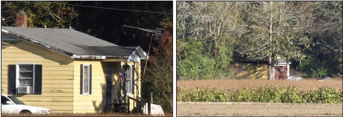
Photo 12: House, 166 Walden Way, Porch Detail (Left) and Garage, South Oblique (Right).
