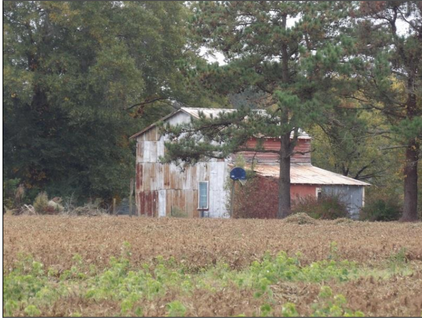
Photo 57: Tobacco Barn, 2290 Davis Homestead Road, Northwest Oblique.
