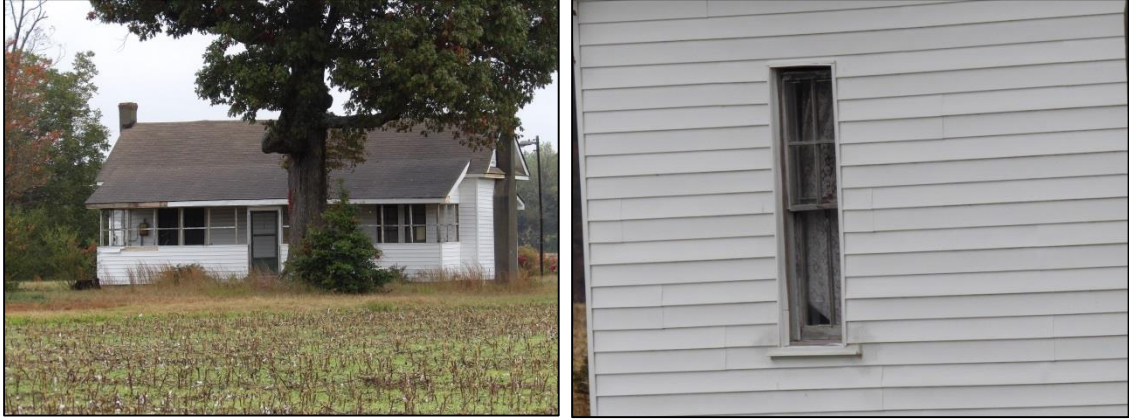
Photo 35: House, 5204 Ringwood Road, South Elevation (Left) and Window Detail (Right).
