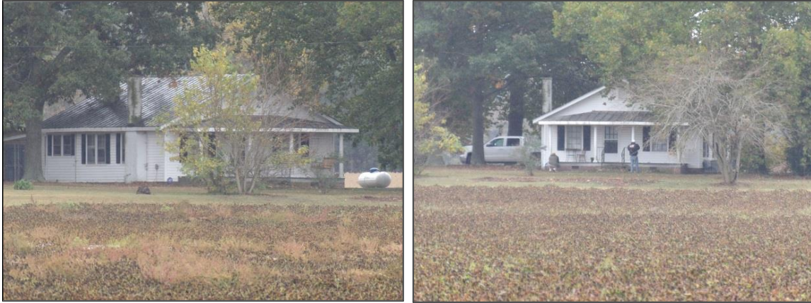
Photo 38: Lee May House, Northwest Oblique (Left) and West Elevation (Right).
