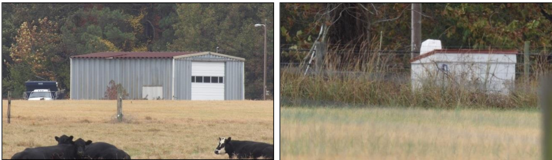
Photo 27: House, Grapevine and Gregory Farm Roads, Garage, Southeast Oblique (Left) and Well House, Southeast Oblique (Right).
