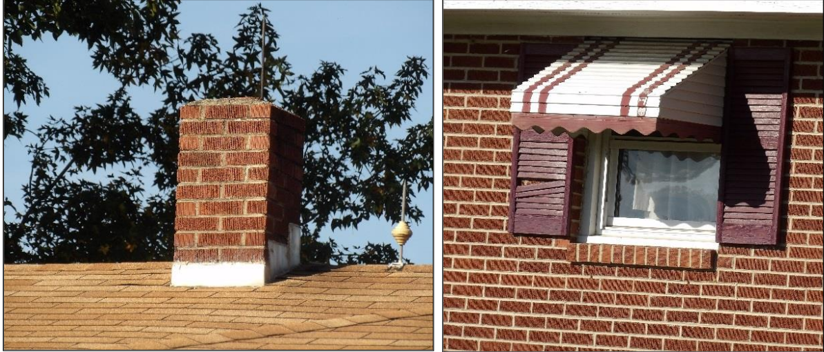
Photo 8: House, 2051 U.S. Highway 301, Chimney Detail (Left) and Window Detail (Right).
