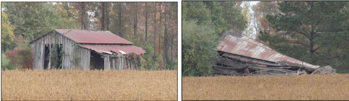
Photo 25: Agricultural Outbuildings, 18656 N.C Highway 561, Looking Northeast.
