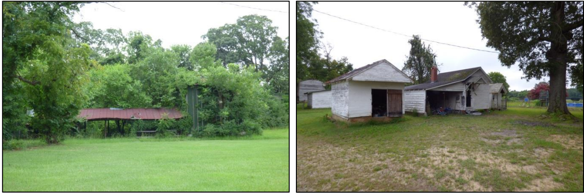
Photo 45: Tobacco Barns, 4170 East Old Spring Hope Road, West Elevations (Left) and Meat House, Summer Kitchen, Well House, West Elevations (Right).
