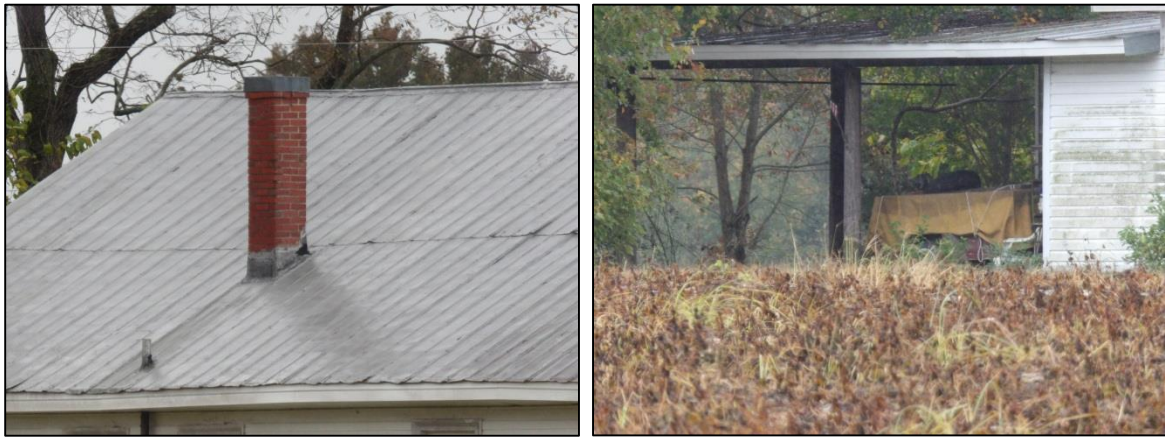
Photo 40: House, 3011 Big Jim Road, Chimney Detail (Left) and Shed-Roofed Addition (Right).
