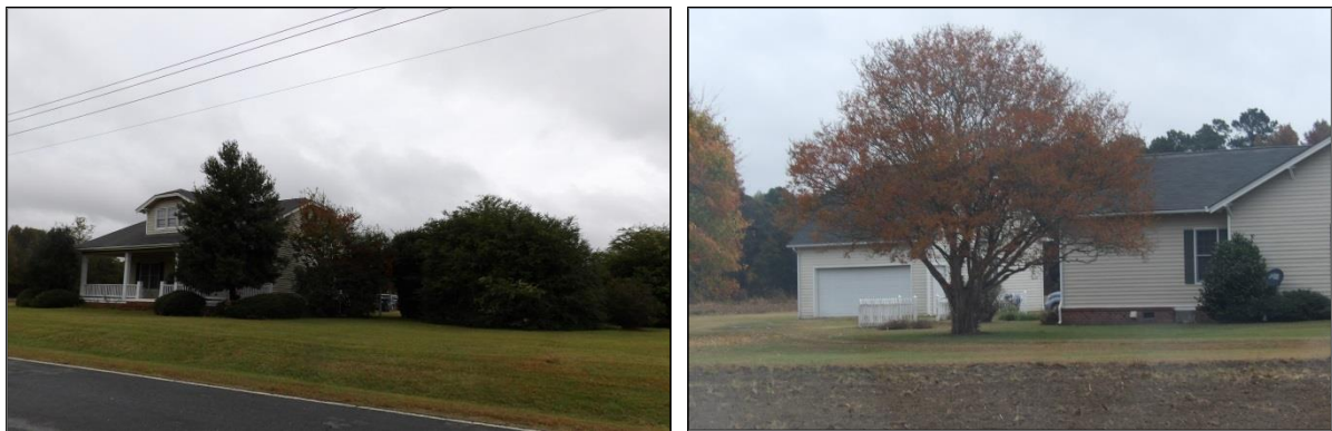
Photo 51: House, 4611 Old Beulah Road, East Oblique (Left) and Garage, Southwest Elevation (Right).
