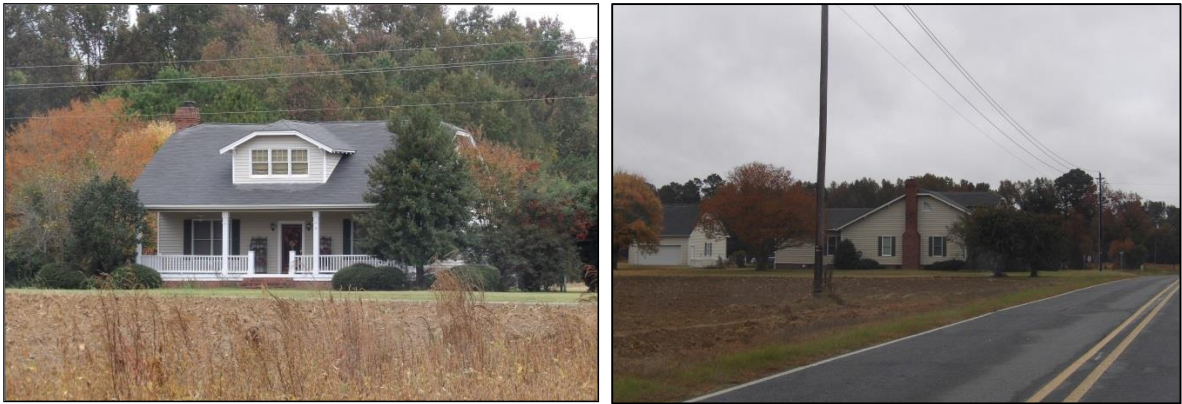
Photo 50: House, 4611 Old Beulah Road, Southeast Elevation (Left) and Southwest Elevation (Right).
