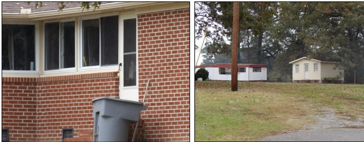
Photo 17: House, 106 Grant Street, Southwest Elevation, Secondary Entrance Detail (Left) and Mobile Home and Shed (Right).
