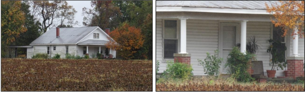
Photo 39: House, 3011 Big Jim Road, North Oblique (Left) and Porch Detail (Right).
