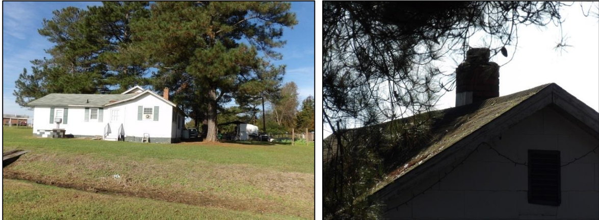
Photo 2: House, 2084 U.S. Highway 301, Southeast Elevation (Left) and Chimney Detail (Right).
