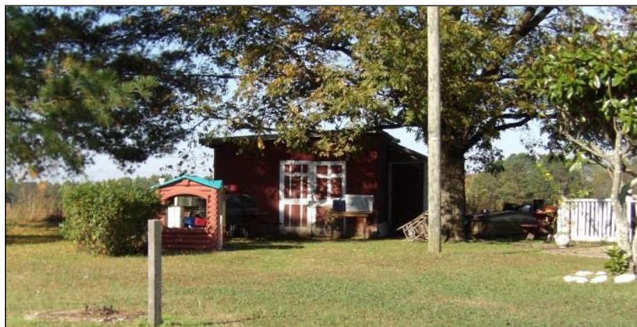
Photo 6: Shed, 2069 U.S. Highway 301, Northeast Oblique
