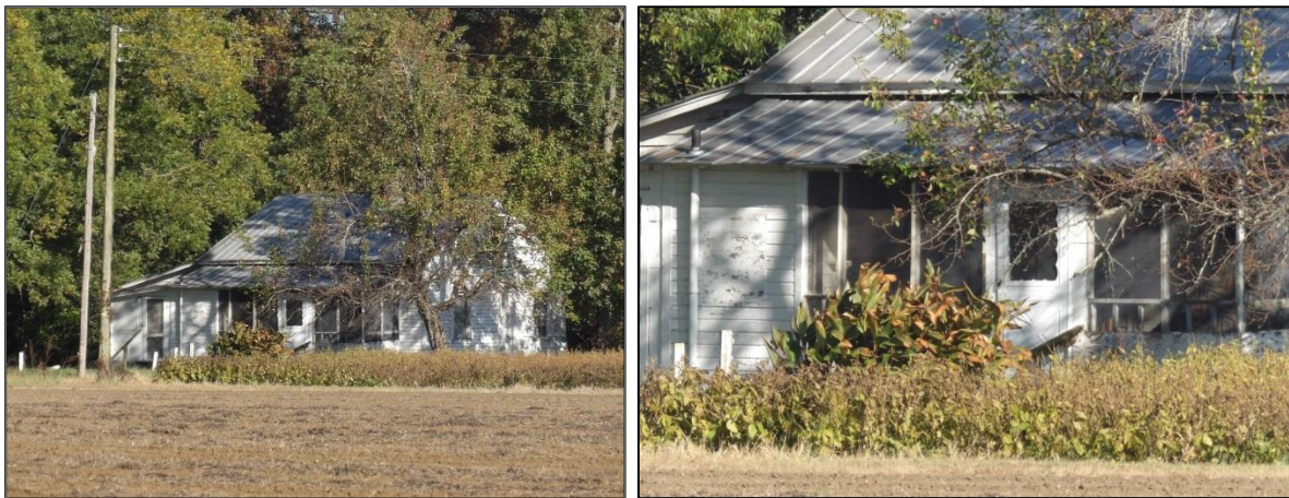
Photo 9: House, 213 Walden Way, South Oblique (Left) and Porch Detail (Right).
